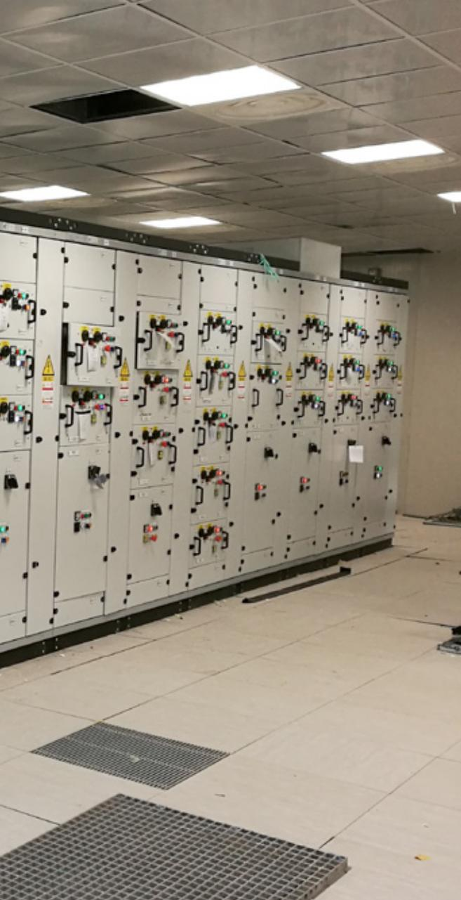
*Fig. 1 – The Power Motor Control Center*
